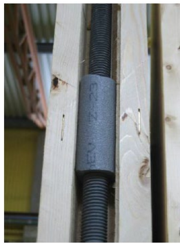
Figure 112 Isolating the post-tension rods in the timber framed walls
