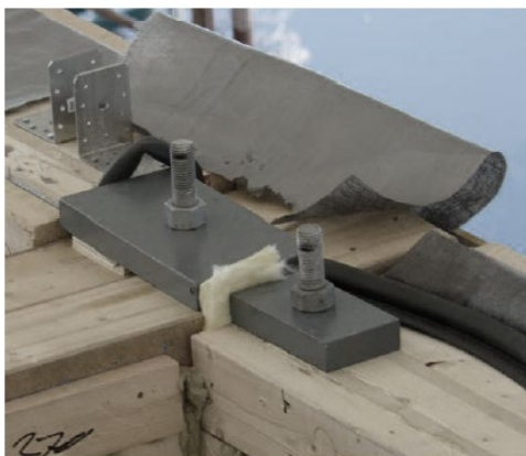
Figure 49 Anchorage of the PT bars at highest point in the Limnologen Project [51]
