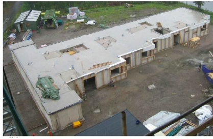
Figure 110 Concrete bottom floor for enhancing the stability
