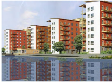
Figure 39 South Façade Limnologen [43]
