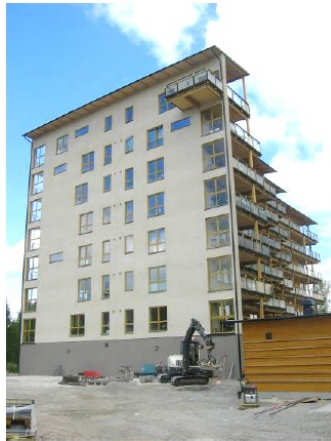
Figure 105 South Façade Limnologen
