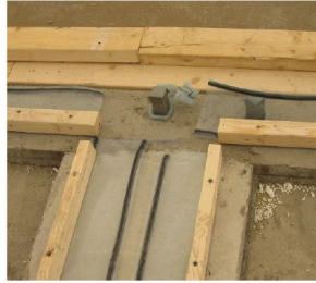
Figure 111 Tie-rods cast in the concrete floor at ground-level
