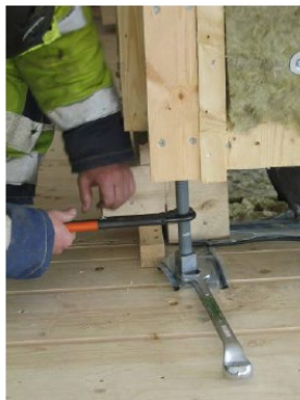
Figure 113 coupling two tie-rods at intermediate height
