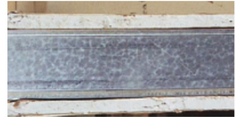
Figure 8 : Gypsum board on metal stud (Binggeli, 2008)
