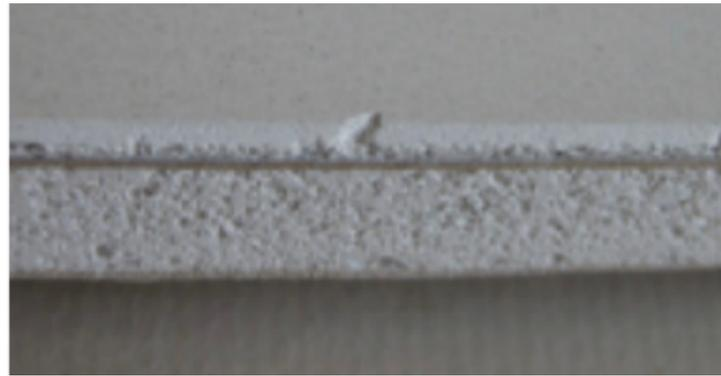
Figure 7 : Veneer plaster on gypsum base (Binggeli, 2008)
