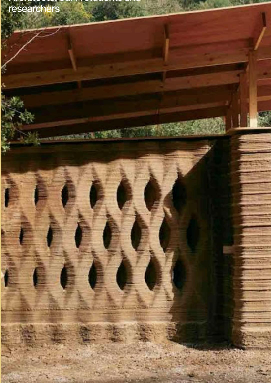
Figure 15: TOVA: 3D Printed Prototype Using Earth (IAAC, 2024)
