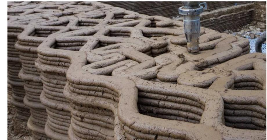
Figure 19: 3D printing wall (Arquitectura Viva, 2024)
