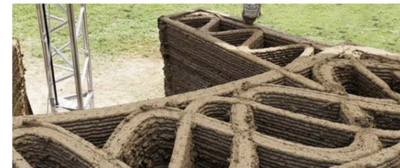
Figure 22: Infill wall (WASP, 2024)
