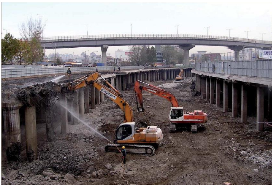
Figure 21 Demolition of the concrete deck of the 10-lane highway
