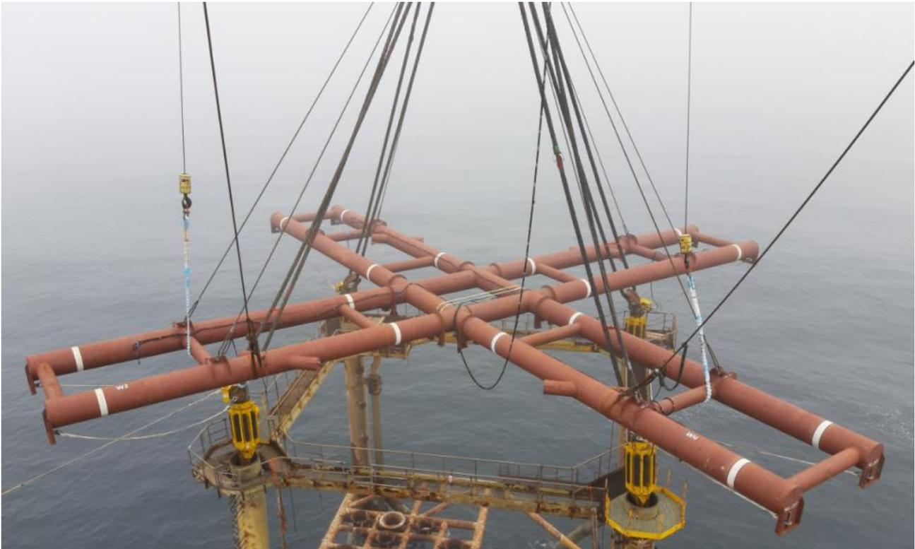
Figure 3.16: The final spacer frame for the V&V 2020 campaign
