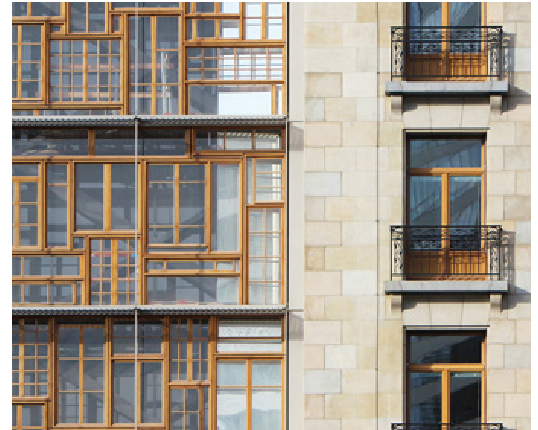
Fig. 22 The oak-framed facade shows the reunion of old and new (Olbrechts, 2016)
