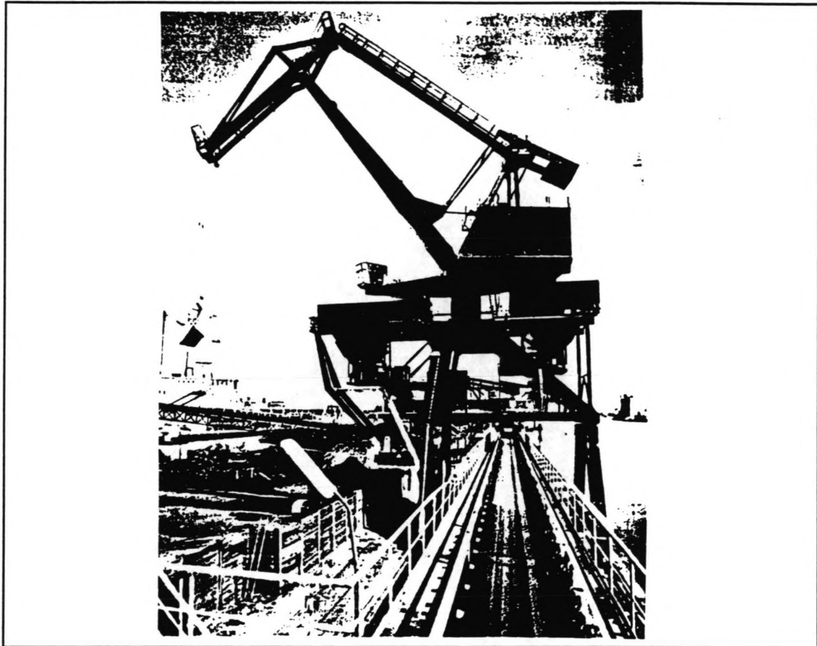
Figure 8.3 portal grabbing crane
