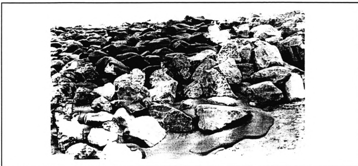
grouted stone coverlayer
