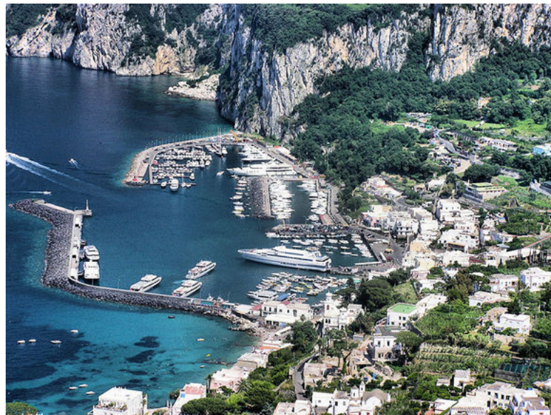
Figure 1.1: Breakwater protecting small harbor, Capri Harbor, Italy
