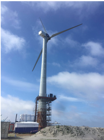
Figure 2-20: Photo display of DOT500 test set-up during prototype testing.
