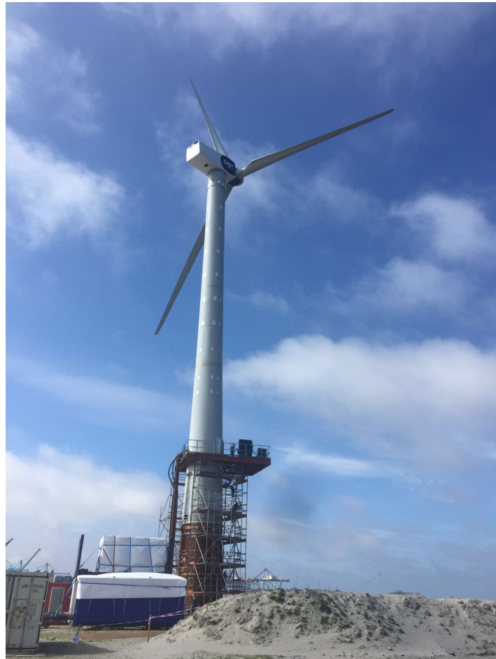
Figure 1: Photo of the DOT500 prototype at Maasvlakte II, the Netherlands.
