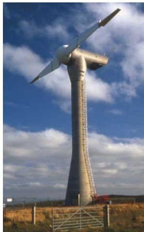
Figure 2-8: Orkney LS1 wind turbine with concrete tower, 1982 [14]
