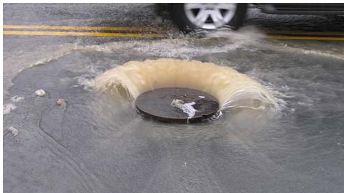
NEW YORK CITY COMBINED SEWER OVERFLOW
