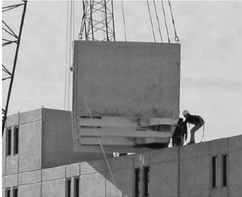
**Figure 9.** Installation of a precast concrete module (Oldcastle Infrastructure).
