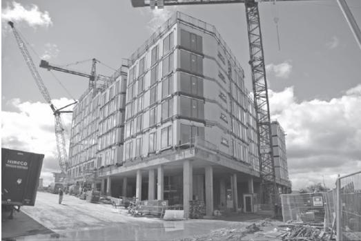
Figure 97. Installation of modules at the Allegro project (Lawson et al., 2010).
