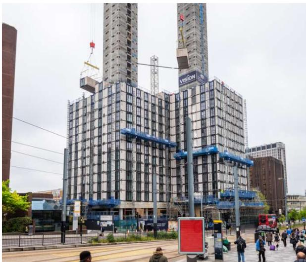
**Figure 78.** Croydon Tower installation of modules (Tide Construction).
