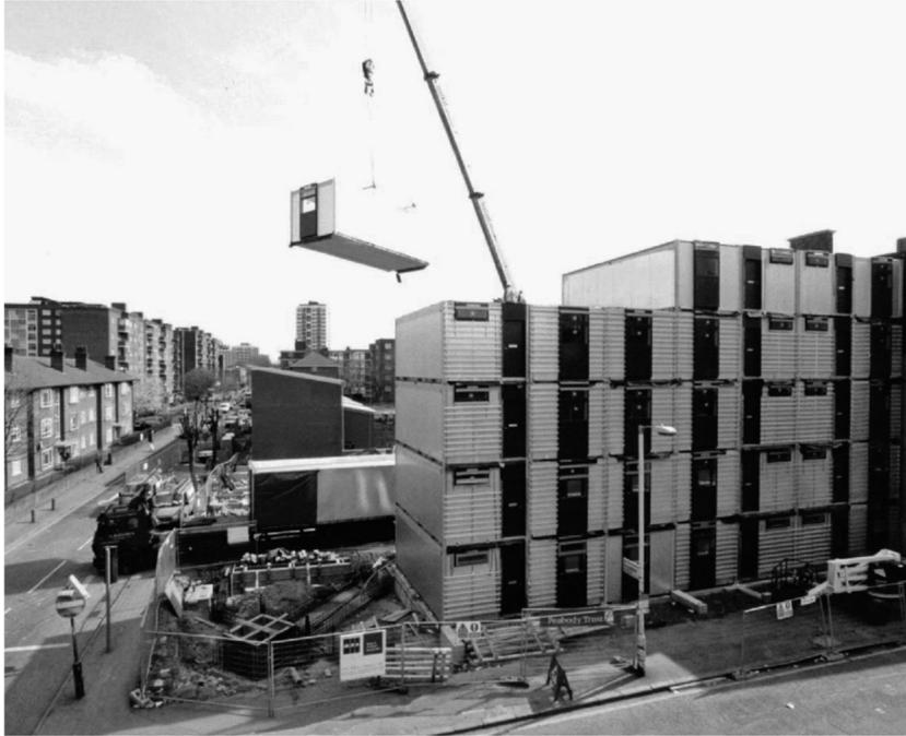
**Figure 1.** Installation of modular units (Courtesy of Yorkon and Cartwright Pickard architects).
