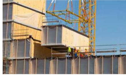
**Figure 12.** Installation of module with CLT walls (Ursem).
