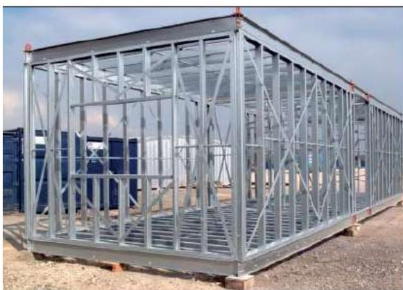
**Figure 15.** Closed module with bracings in both directions (Lawson et al, 2005).
