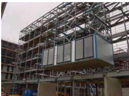
**Figure 92.** Braced walkways of MoHo (Steelconstruction.info).
