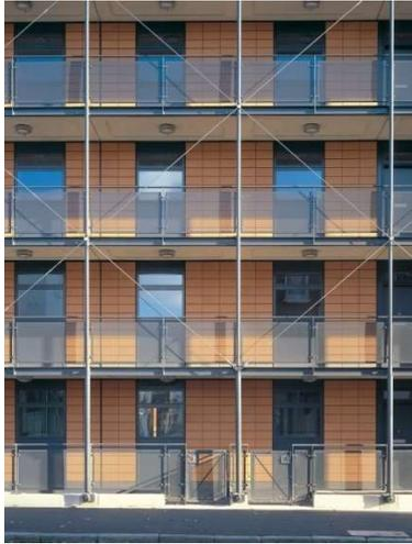
**Figure 87.** Braced access walkways of Murray Grove (Cartwright Pickard).
