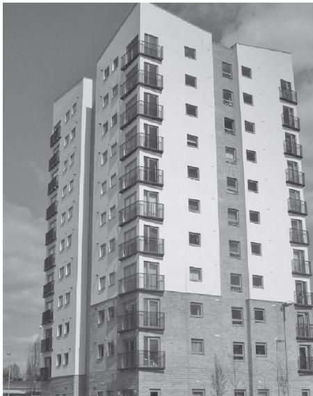
**Figure 82.** Eleven-storey modular building, Basingstoke (Lawson et al., 2010).
