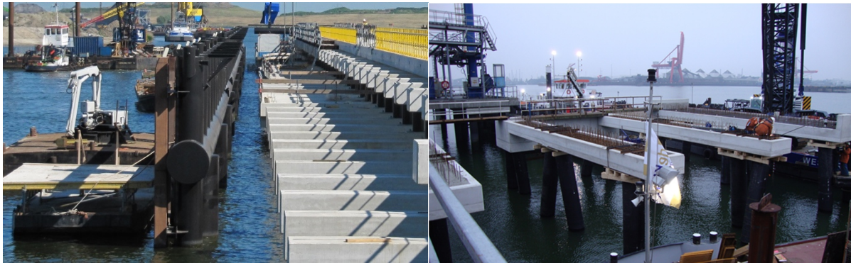
Figure 9: Left: Main freestanding flexible dolphin (SBRCURnet, 2018a); right: tubular piles with prefab beams (SBRCURnet, 2018b)
