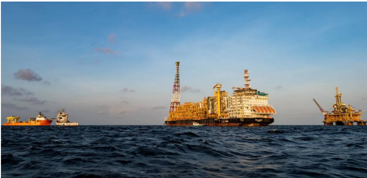
Figure 1.1: A field production unit in its operating environment
