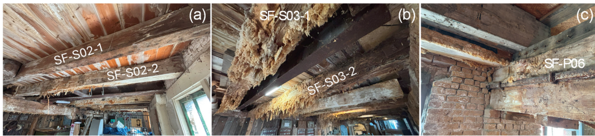
Figure 9. (a) beams assessed at the 2nd floor of Lijfland building, in the first span showing limited signs of defibration. (b) beams located on the 2nd floor in the mid bay, showing extensive signs of defibration. (c) detail of the connection between masonry wall and primary beam SF-P06.
