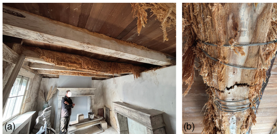
Figure 3. Effect of crystallization in timber beams (a) leading to the rupture of a secondary timber beam (b) on the ground floor.
