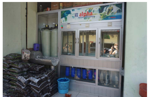
Figure 26 A store in kampung Kandri where water is being treated with UV radiation to be of drinking water quality.
