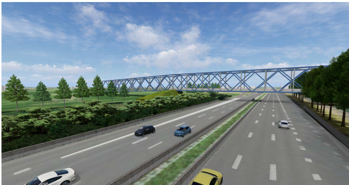
Figure 8.2: 3D render design for Ackerdijksebrug based on three 100-m bridge objects from donor Keizersveerbrug.
