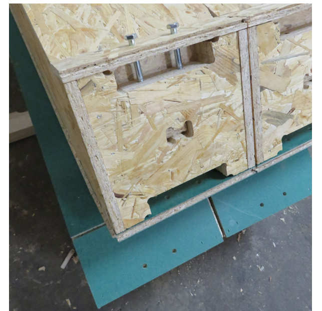
Figure 9.12 a) The top connection of two roof blocks and b) inserted joint, rubber and tongue/groove edge to make firm, air and watertight structure (Own illustration)
