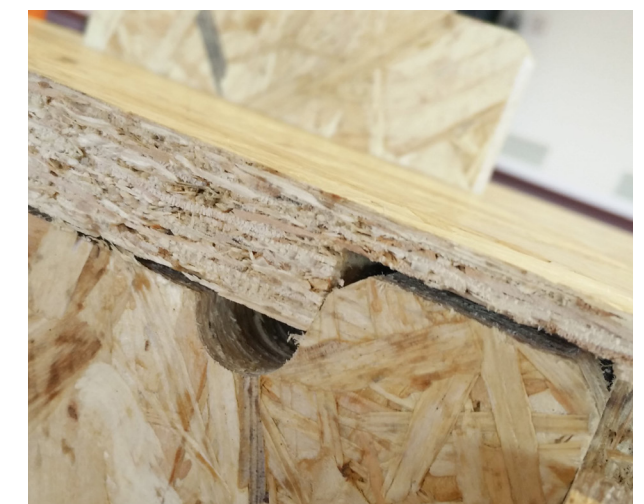
Figure 8.10 More process time required to close the rounded openings (Own illustration)
