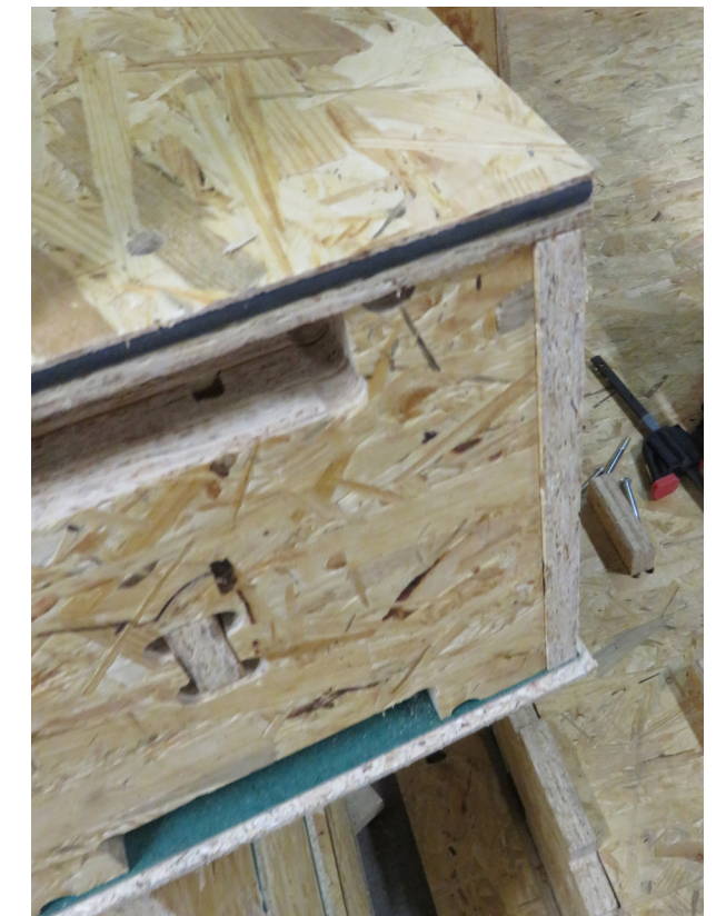
Figure 9.4 Integration of air and water tightning in a component due to the ability to produce with low tolerance (Own illustration)
