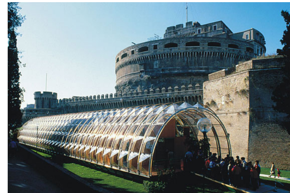
Figure 3.11 Renzo Piano pavilion (1983) is one of the early projects adapting design for disassembly principles (rpbw.com)
