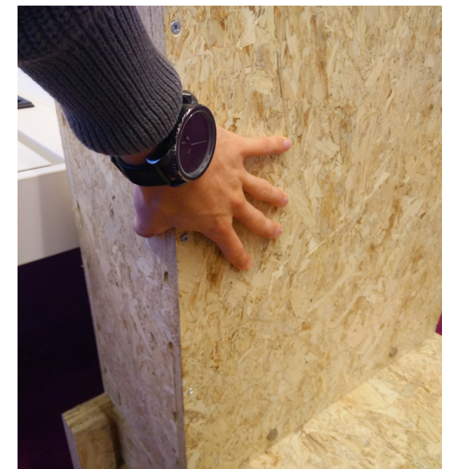
Figure 8.21 a) Trouble getting grip on the wall components and b) floor components can be lifted with the bolts (Own illustration)
