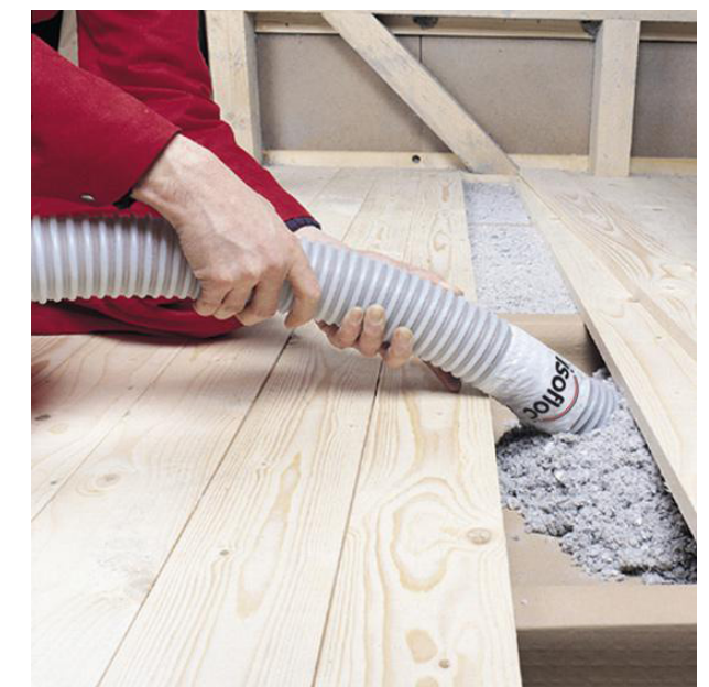
Figure 6.9 Applying cellulose insulation (isofloc.com)
