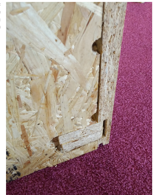
Figure 8.7 Inaccuracies resulting in gap between the different elements (Own illustration)
