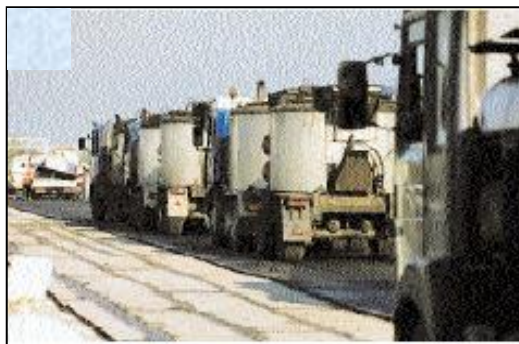
Figure 3.3: Isolated transport of mastic asphalt
