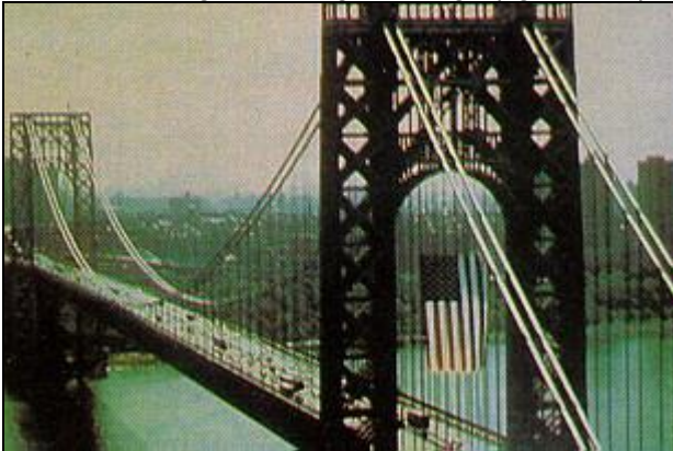
Figure 3.30: George Washington Bridge
