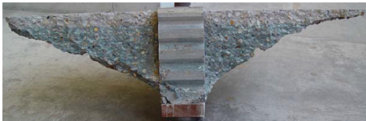
Figure 2.6: Punching shear cone element after failure [16]
