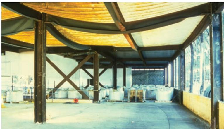
Fig.2.7. Cardington: overall frame deformation after a fire [37].
