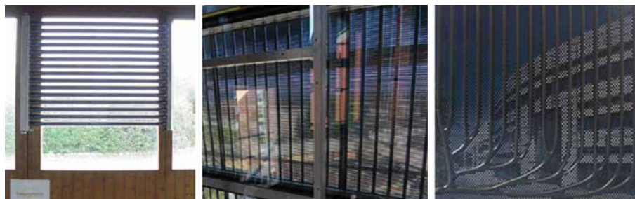
FIGURE 8.61 Three images left: examples of thermal solar collectors with semi-transparent façade. Right: Spuiplein and Theatre, The Hague.
