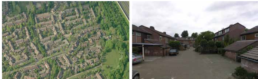
FIGURE 8.32 Example of low strips and open urban blocks with little to moderate green, in Maarsse.
