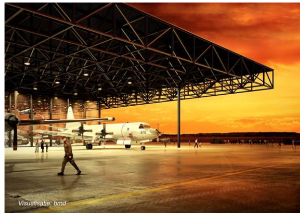
Figure 2.2: Application of structural optimisation on a space-truss. The goal of optimisation in this project: "Nationaal Militair Museum Soesterberg", was to minimise the weight of a 8000 element truss. The result was a 60 \text{ kg/m}^3 roof instead of the 100 \text{ kg/m}^3 which is usual for these kind of spans. The engineer in this project is ABT [8]. Courtesy: ABT [8]
