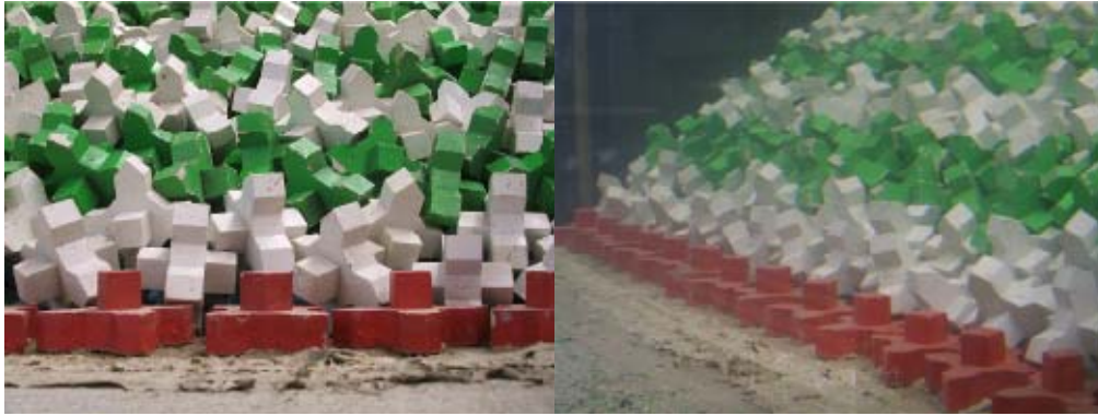
figure 3.10: Toe construction with Xbase units
