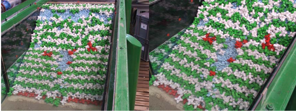
figure 3.20: Failure of the armour layer and exposure of the first under-layer
