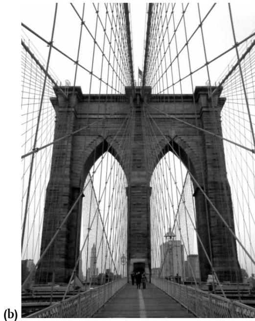
Figure 6.1: (a) Main components and characteristic dimensions of suspension bridges. Based on (Harazaki et al.: 2000) (b) A view of John Roebling's Brooklyn Bridge in New York showing his trademark diagonal cable stays radiating from the top of the tower. See main text for details.
