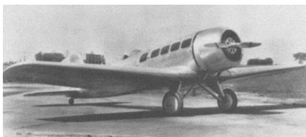
Fixed tripod landing gear on a Northrop Alpha
