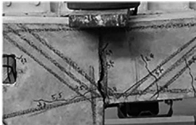
(c) Actual failure of specimen G-1 [19]
