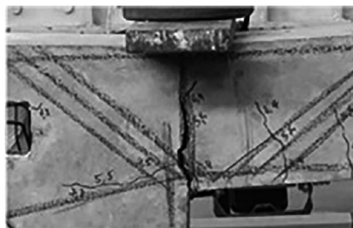
(c) Actual failure of specimen G-1 [19]
