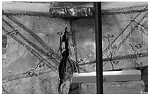
(c) Actual failure of specimen H-1 [19]
