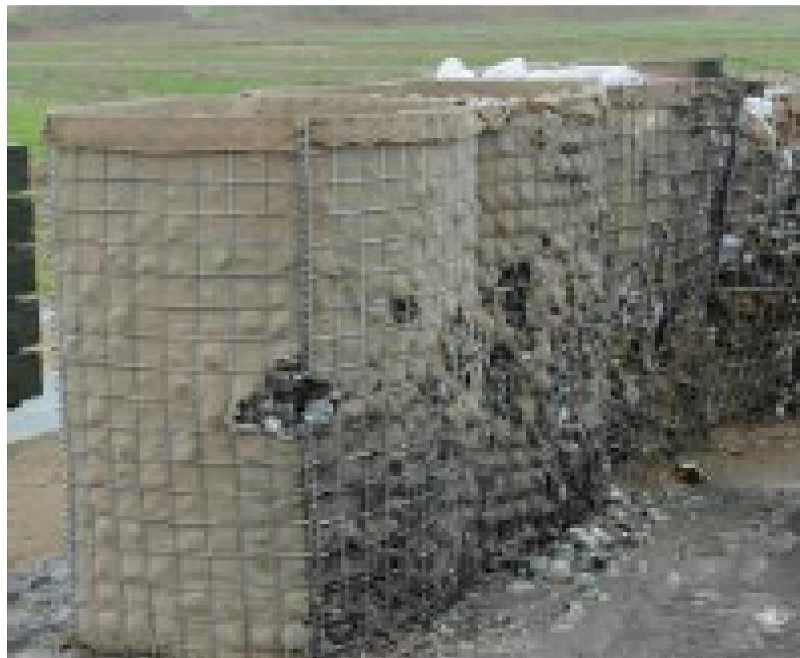
(a) Cobble filled wall
