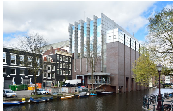
Current exterior of backstage Carré
