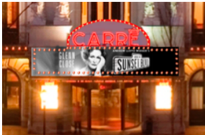
Marquee on front façade
