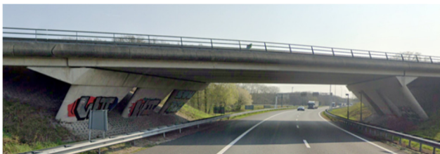
Motorway viaduct 'Grollegat'
