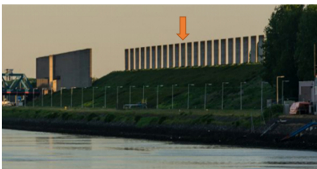
Wind deflecting structure Caland channel
