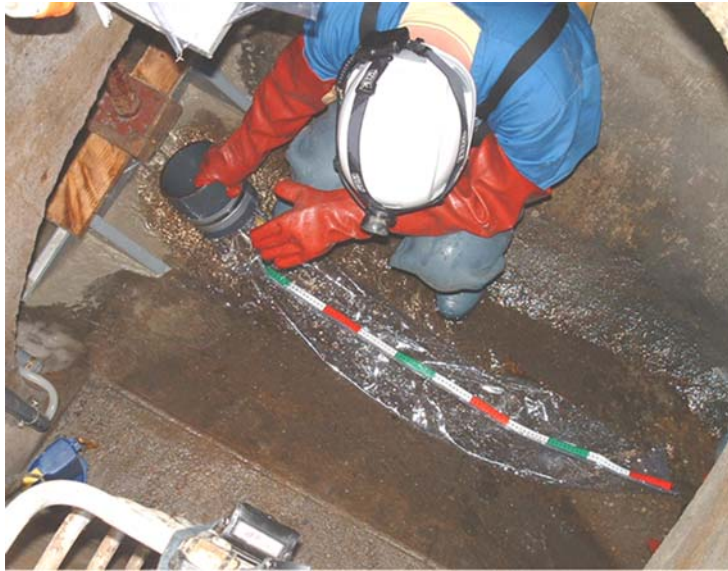
Figure 3.1 Implementation of a device to capture all the volume flowing through a weir. Source: Université Gustave Eiffel.
