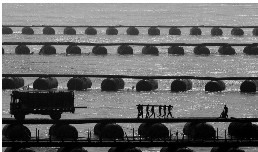
Wooden planks are then laid and fastened to the girders.
