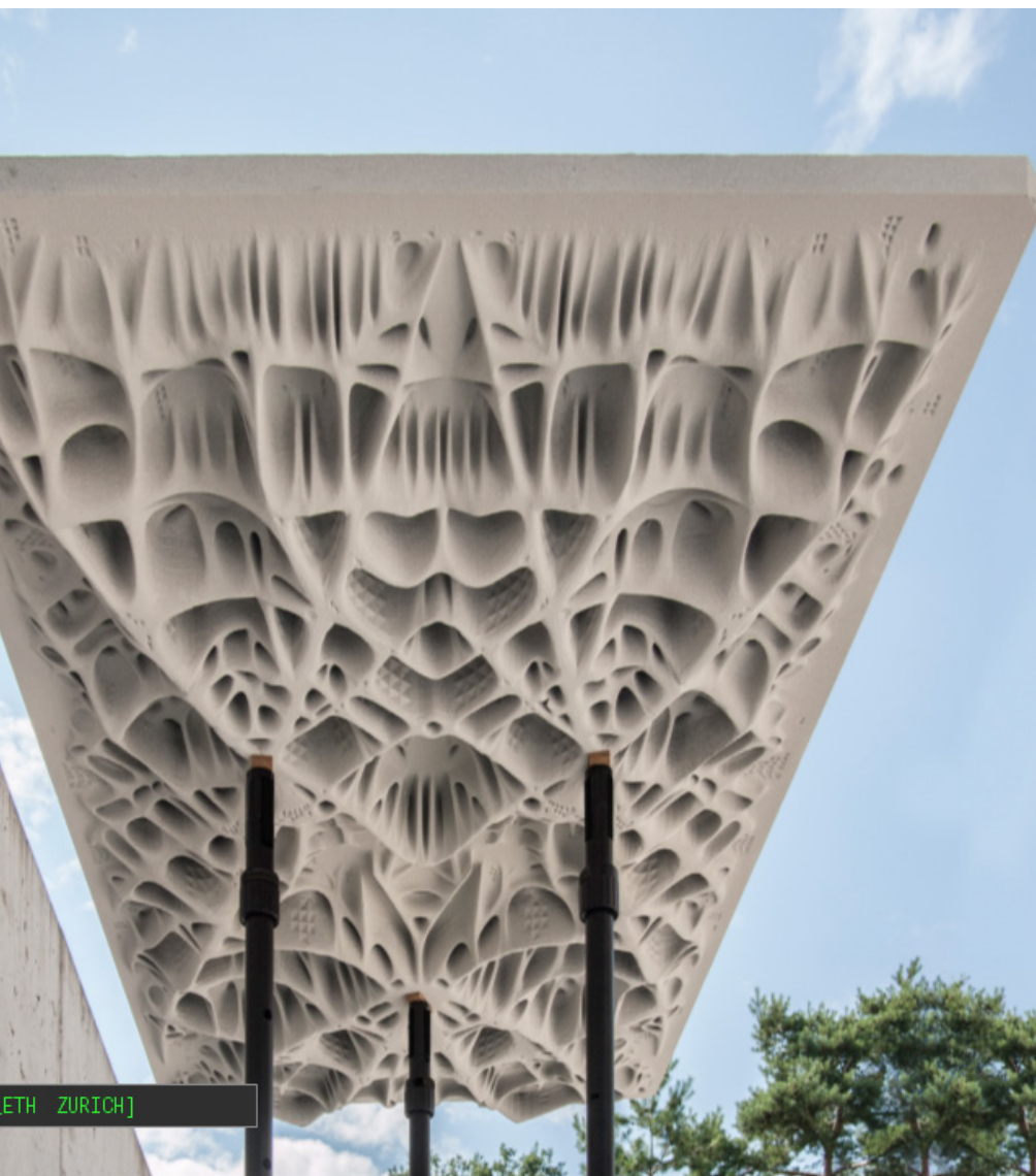
Smart slab project at ETH-Zurich using the powder bed production technology
