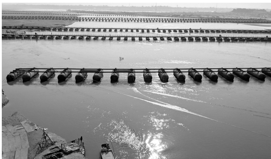
Once in position, steel girders are laid on top to anchor each pontoon together.
