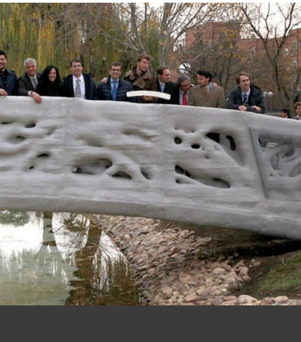
D-Shape projects using powder bed 3d printer. The first pedestrian bridge printed in 3D in the world in the urban park of Castilla-La Mancha in Alcobendas, Madrid.
