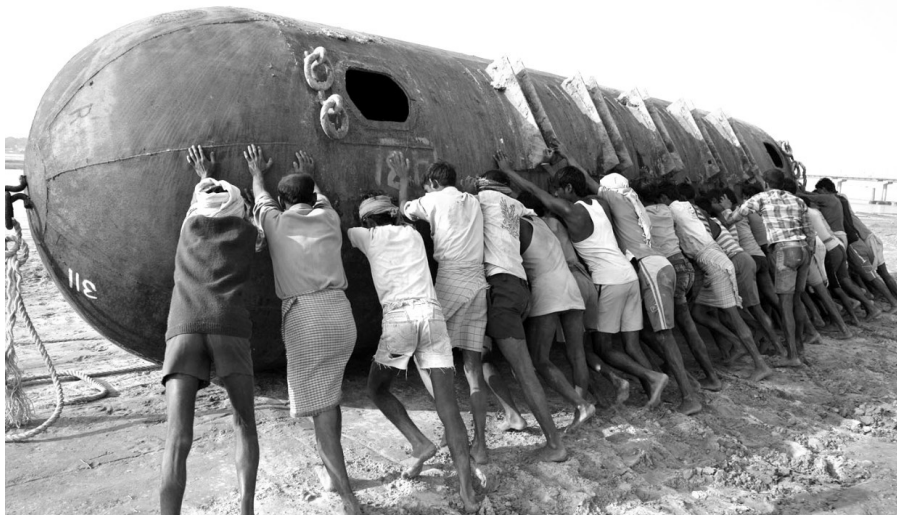
The bridges are constructed off-site, transported to site and then manually put into position in the water.
