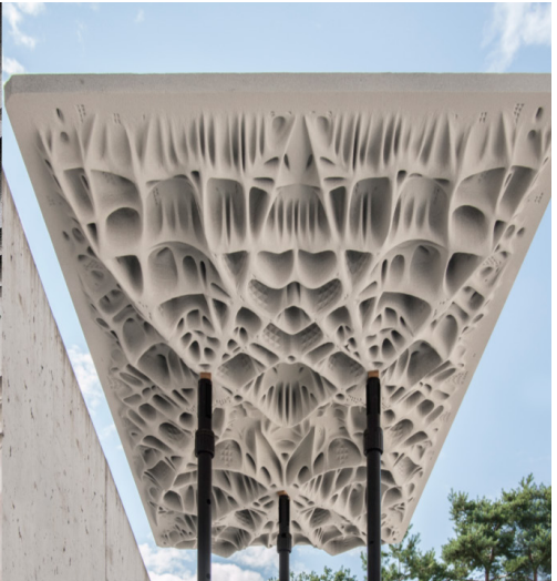
Above Image : D-Play Bottom Image: Smart Slab. Eth-Zurich Particle bed 3d printer used for production
