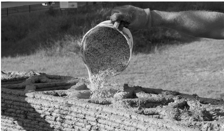
Technique: HI-Tech/Crane Wasp Material: Clay, Silt, Sand, Straw & Husk Binder: lime Coating: shaving claylaminallinseed oil
