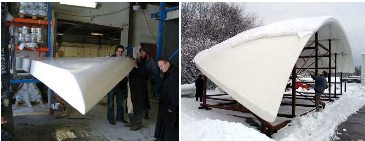
Fig. 28-29. Roof segment (left) and fitting of all the roof segments of the lower wing of 'The Library' at Holland Composites in March 2005.
