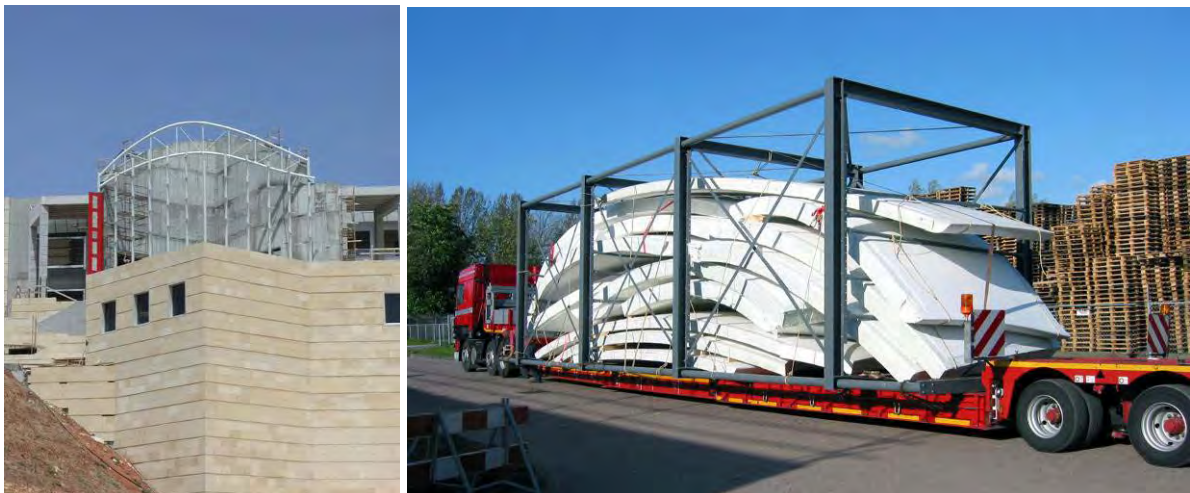
Fig. 30-31. Building site in Tel Aviv zoomed in on 'The Library' with the truss and columns already installed (left). Open container at Holland Composites with the roof segments ready for shipment in April 2005.
