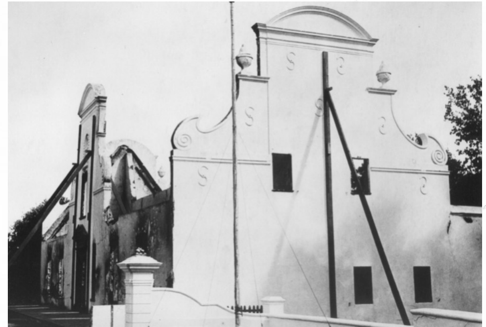
Figure 22 - Depiction of the reconstruction of Groot Constantia's primary homestead after the 1925 fire. British architect Franklin Kendall led the project. He focused on restoring the building to as close to its original Cape Dutch style as possible, rebuilding the thatch roof that caused the fire to rapidly spread.
