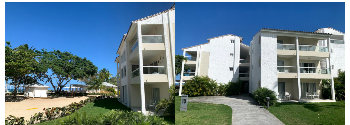
Figure 51: Side and Frontal views of Guest Block 16. Source: own
