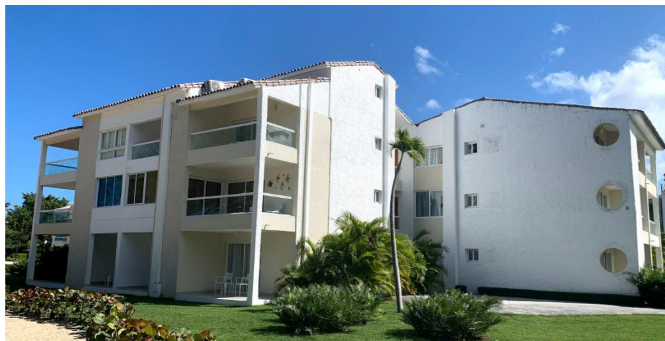
Figure 52: North view of Guest Block 16. Source: own
