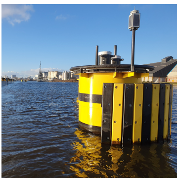
(a) Mooring dolphin with a bollard
