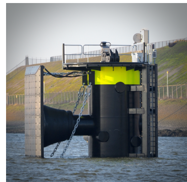
(b) Berthing dolphin with a fender
