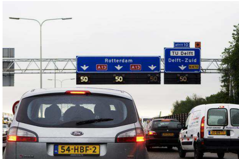
Figure 1-2: Example of infrastructure that is used to impose variable speed limits in The Netherlands. Source: taxipro.nl
