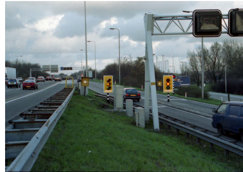
Figure 1-3: Example of infrastructure that is used for ramp metering in The Netherlands. Source: commons.wikimedia.org
