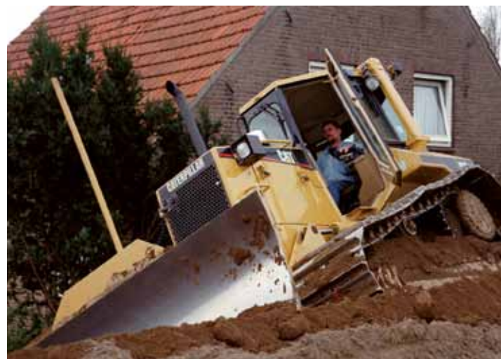
Dyke reinforcement using heavy equipment.
