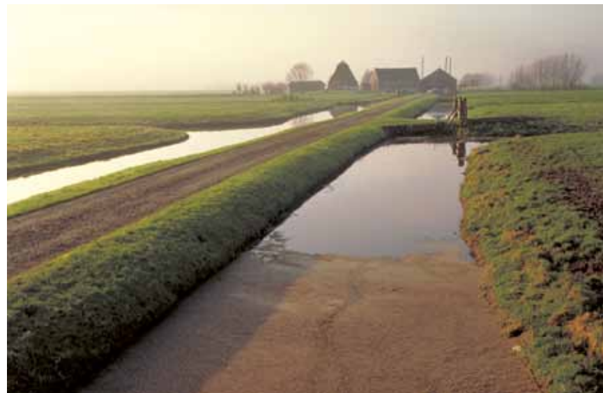
Schenkelkade, a low peat dyke that functioned as a boundary in the Krimpenwaard near Haastrecht.
