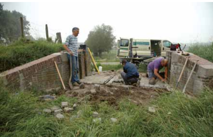
Restoration of a cut in the old dyke between the Nieuw-Westenrijk and Van Wyckhuise polders in Hoek (Zeeuws-Vlaanderen). Supervised by a contractor, volunteers from the Stichting Landschapsbeheer Zeeland restore the paving of the cut.
