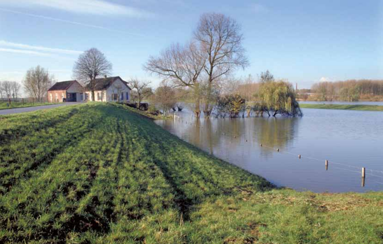
High water along the Rijnbandijk at Maurik, with the flood plains submerged. The low summer dyke can be seen on the right behind the trees.
