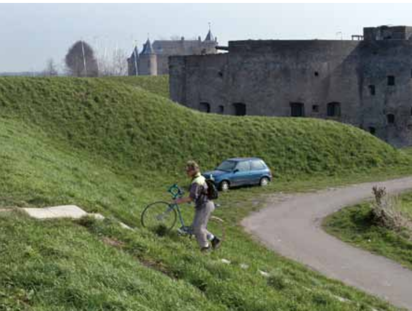
Zuiderzeedijk at the West Battery fort in Muiden.
