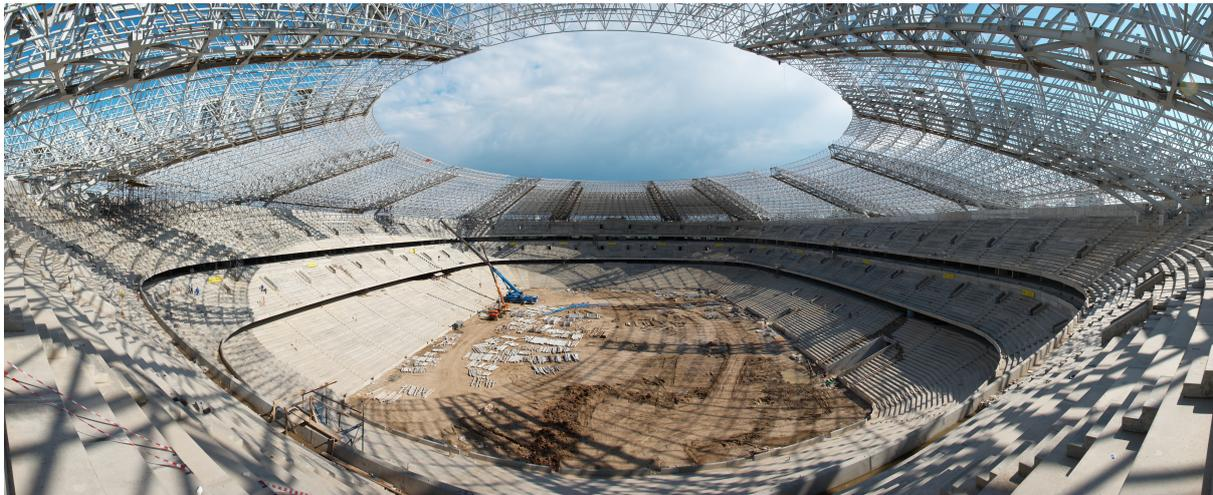
Figure 5.2: Roof structure of Donbass Arena during construction (Academic, 2014)
