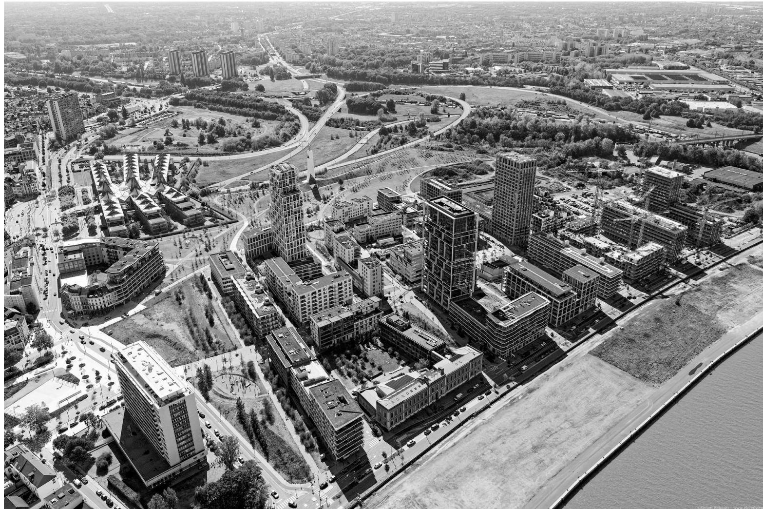
New South under construction
