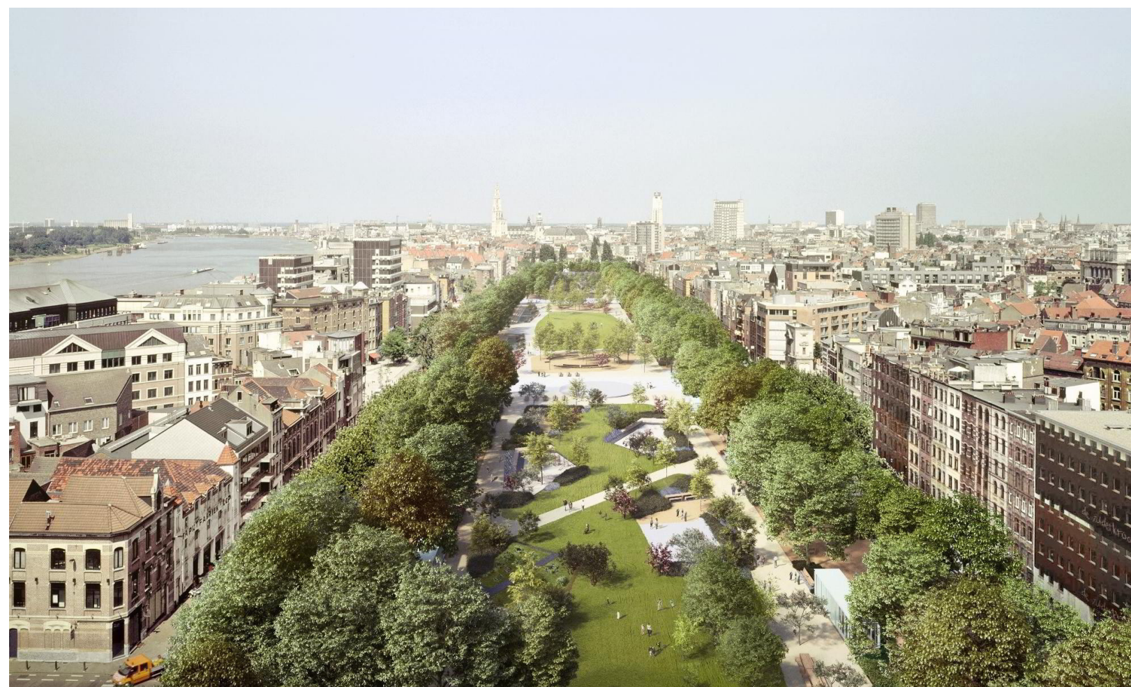
Development of New Park in the former dock
