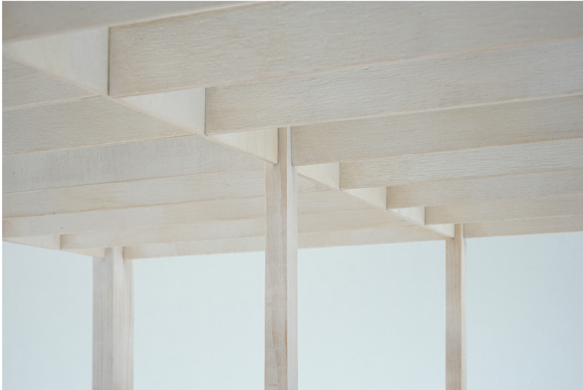
Primary Timber Structure – Glue-Laminated Columns and Beams
