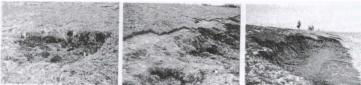
Figure 10.2 Damages on the outer slope at highest tide water level during storm flood of February 1962, Germany. [Pohl, 2006]
