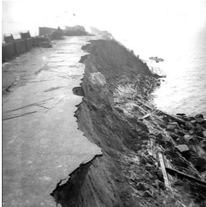
*Figure 10.12 A dike which just did not fail, during the storm surge disaster of 1953. The cliff erosion which developed till the core of the dike can clearly be seen. [www.deltawerken.com]*
