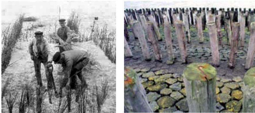
Figure 2.2 Left: Men making mattresses of osier wood ('krammatten') and right: Rows of piles with basalt in between ('staketwerk').
