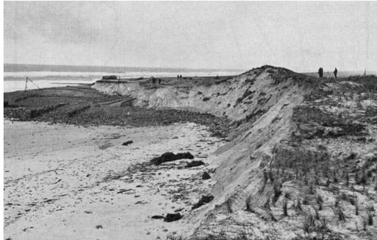
Figure 10.13 Dune erosion at the connection to the Hondsbosse sea defence at Kamperduin. [Rijkswaterstaat, 1961]
