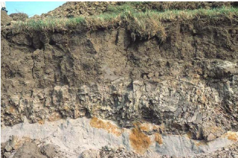
Figure 6.2 Soil structure in a dike. The influence of animal burrowing and root penetration to 0.7m deep. (The structure underneath is a result of changes in moisture content.) [TAW Klei, 1996]
