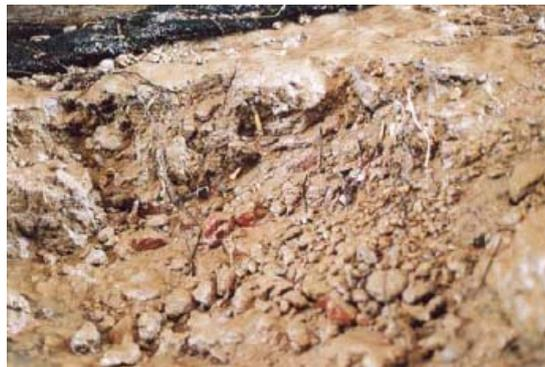
*Figure 4.5 Damage of the clay layer with a soil structure under a stone revetment. The clay eroded in the form of lumps to a depth of 0.4m deep.*
