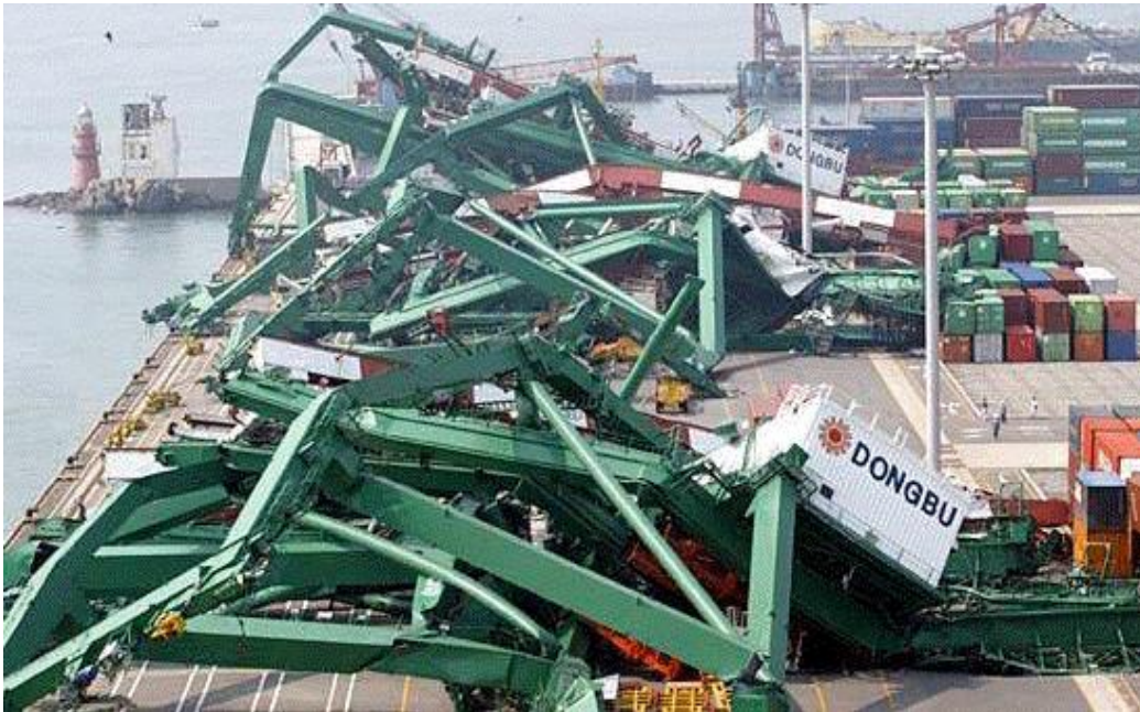
Figure 8.1 – STS crane collapse after typhoon Maemi (up to 215km/h) in Port Busan, South Korea [www.cargolaw.com]
