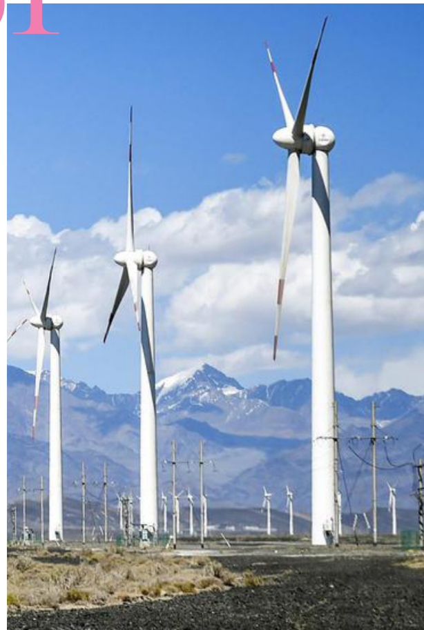
Fig. 3.6, Wind energy Low-carbon energy transition in China. Image source: https://xi.chinadaily.com.cn/a/202204/22/WS62623645a3101c3ee7ad1c9b.html
