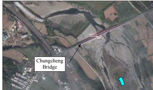
Figure 2. Aerial photo of rebuilt Chungcheng Bridge (taken in 2015).
