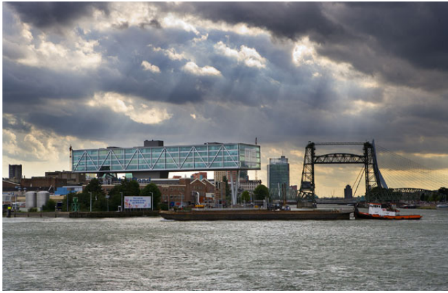
Figure 6.1 Unilever building; foundation and Construction; execution on plot
