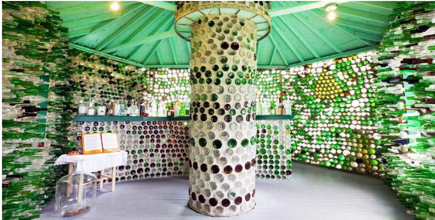
Figure 6 – Circular column Design in The Bottle Houses (Byers, 2018)
