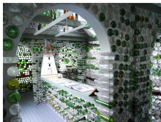
Figure 5 – Column design in The Bottle Houses (Rom, 2015)
