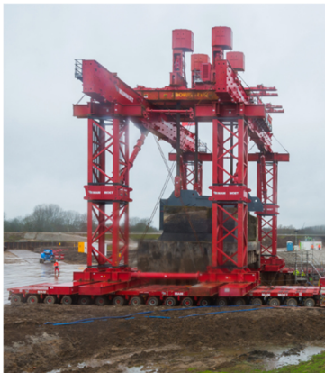
c) Mobile gantry [47]
