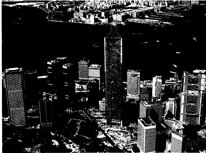
1.28 Hong Kong, Bank of China (nov. '88), hoogte 320 meter architect: I.M. Pei & Partners en Kung & Lee
