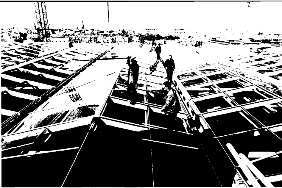
Atriumglaskapbeglazing. project: Stadhuis te Den Haag architect: Richard Meier
