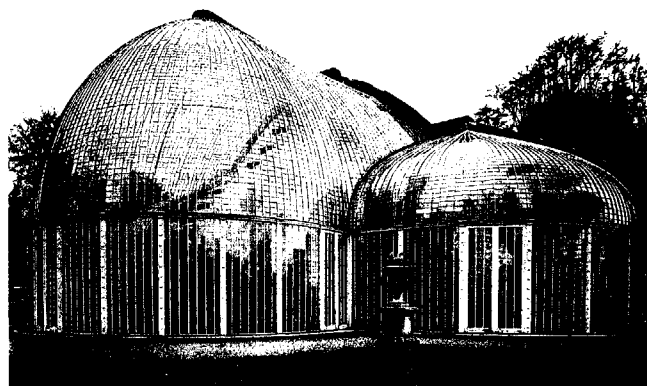
3.88 Palm House, Bickton Gardens (GB), 1818/38. architect: J.C.Loudon
