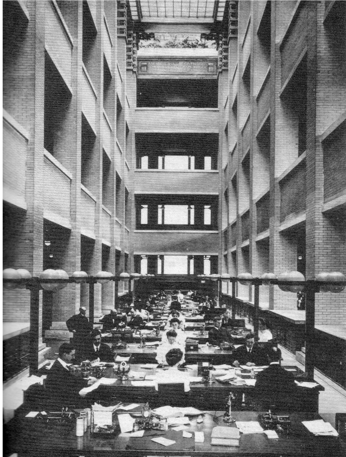
Larkin Building - Frank Lloyd Wright - 1905
