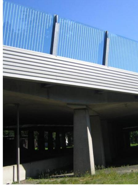
Figure 133 Tapered section at the intermediate support [15]
