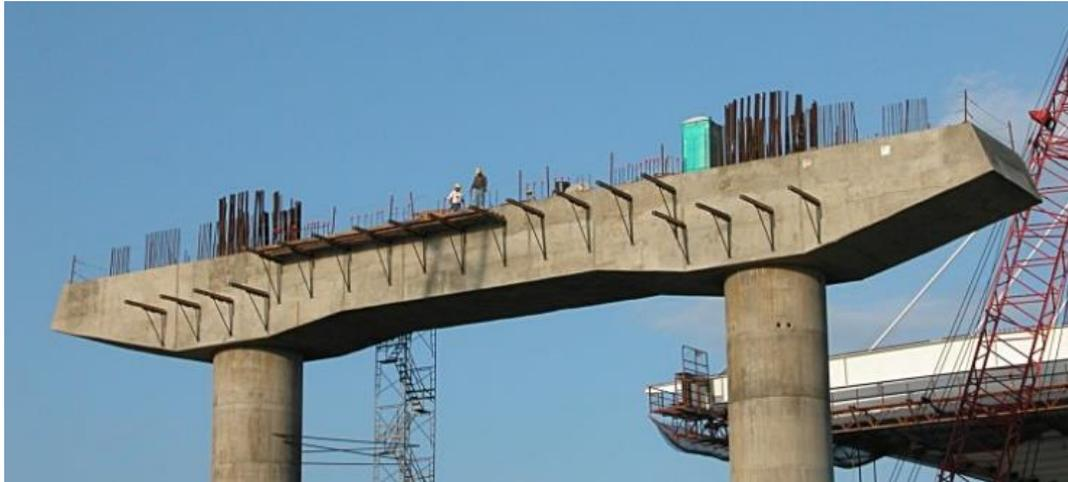
*Figure 1 Haunched capping beam*
