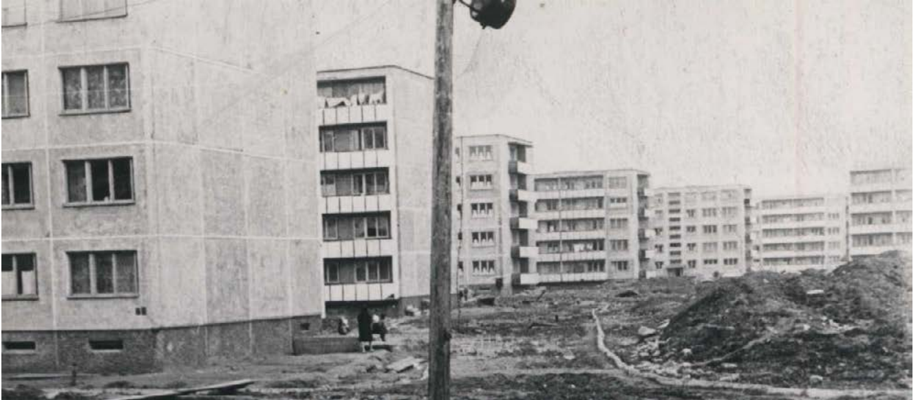
Image: Beginning of Construction in Silainiai (Source: Archive of Kaunas)
