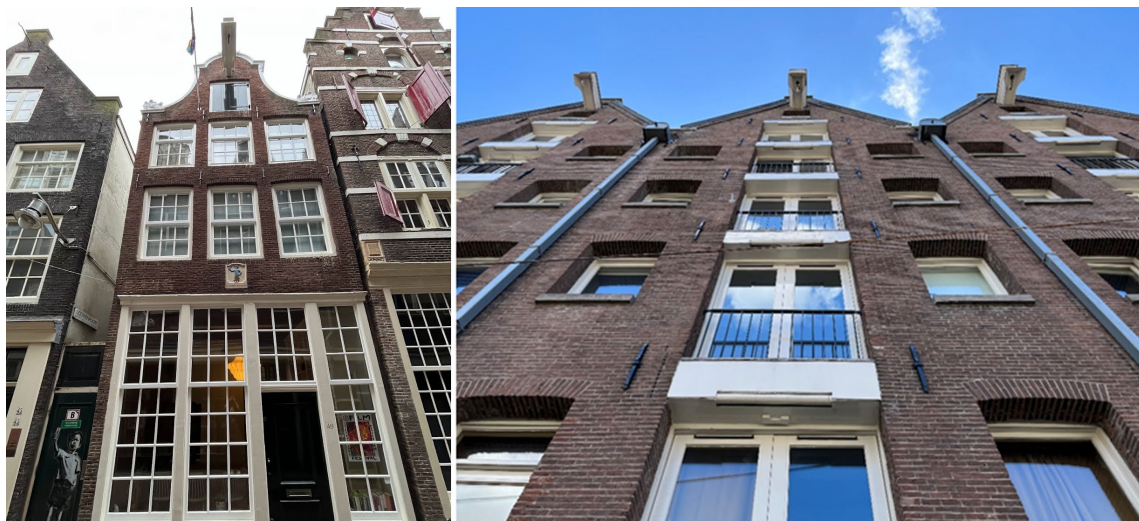
Figure 4. Front facades of the two reference buildings for energy calculation [43].
