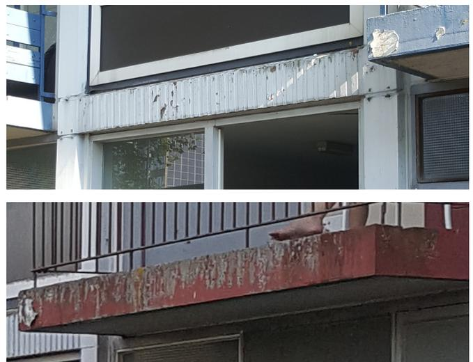
Figure 1.3.6 . Cladding with poor maintenance
