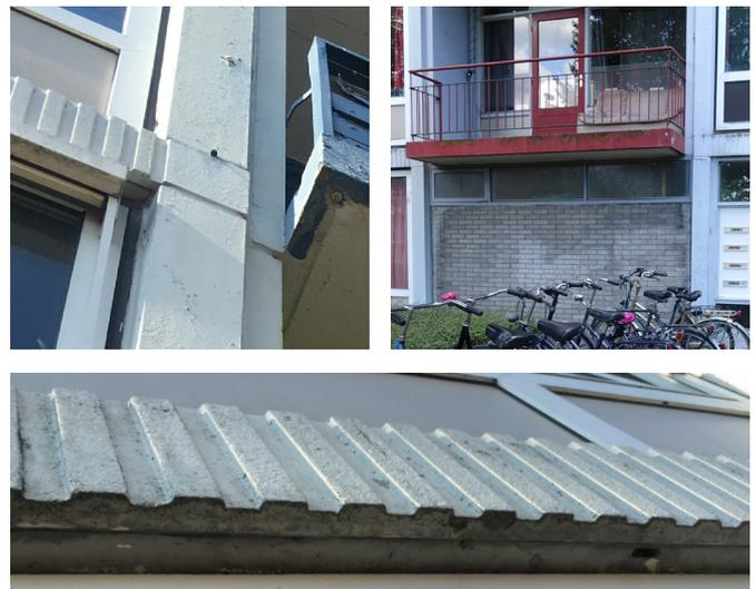
Figure 1.3.5 . Prefabricated fragments attached to structure
