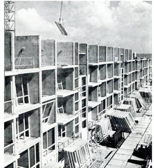
Figure 1.2.3: Assembly on site
