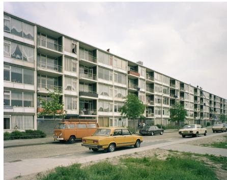
\*Figure 1.3.14. 1984: Timber window frame with Single glazing
